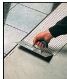
For floor tile application apply the mixed adhesive direct to the floor in a uniform layer 3-6 mm thick. Press the dry tiles firmly into this layer of adhesive to ensure the absence of voids beneath the tiles. Alternatively, trowel the adhesive layer with a trowel having 20 mm notches at 30 mm centres, before pressing home the tiles.
